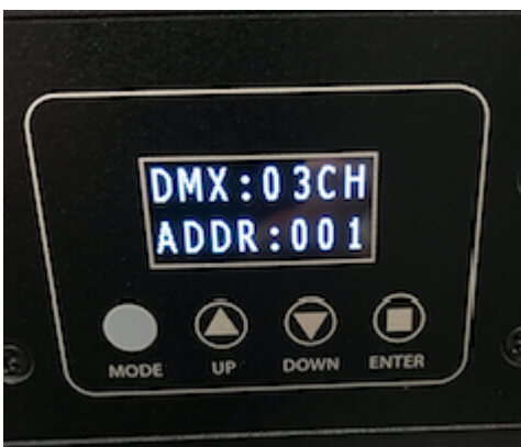
DMX CABLE CONNECTED
