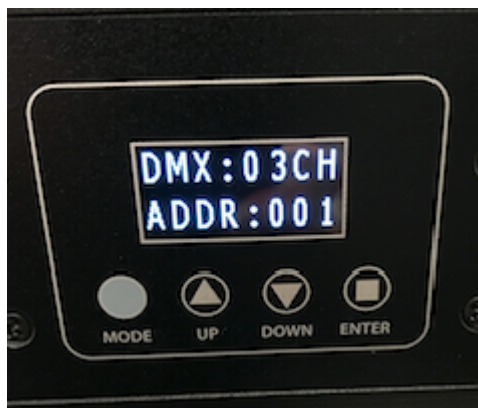
DMX CABLE CONNECTED
