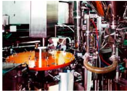
Inspection Lights Control
