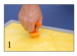
Screw Primacoustic Snap-On Anchors into the back of the panel using the driver tool.
