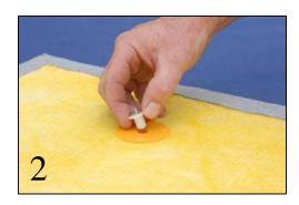
Insert marking plugs into the Snap-On anchors.
