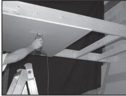
Fig. 5: Cutting drywall using the Rotozip™.
