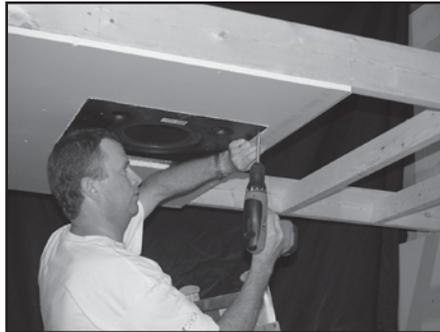
Fig. 8: Attaching the subwoofer to the pre-installation ring.
