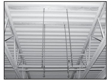
Fig. 13: Suspension points with turnbuckles installed.
