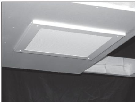
Fig. 10: Completed subwoofer installation.
