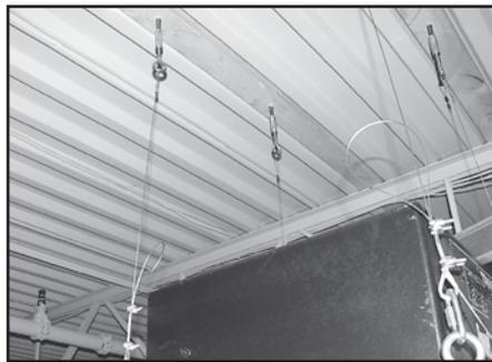
Fig. 15: Eyebolts in place of threaded rod.
