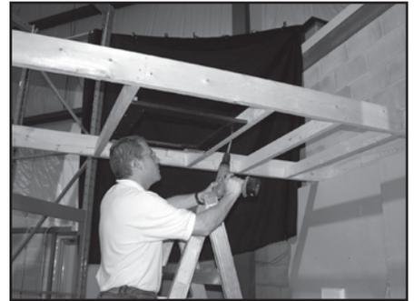
Fig. 3: Attaching pre-installation ring to blocking.
