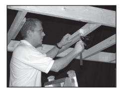
Fig. 1: Installation of blocking for flush mounting of pre-installation ring to joists.
