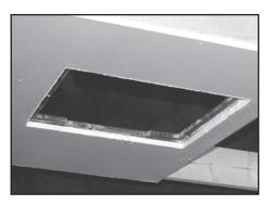
Fig. 6: Completed install showing the reveal of the pre-installation ring relative to the ceiling board.
