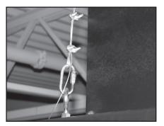
Fig. 8: Wire rope detailing suspension or seismic tether.
