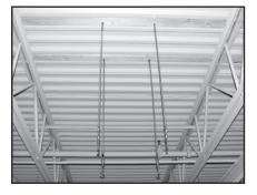
Fig. 13: Suspension points with turnbuckles installed.
