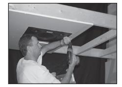
Fig. 8: Attaching the subwoofer to the pre-installation ring.
