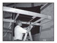
Fig. 3: Attaching pre-installation ring to blocking.
