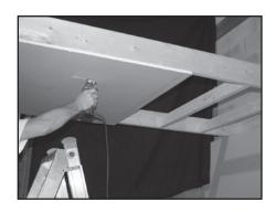
Fig. 5: Cutting drywall using the Rotozip™.
