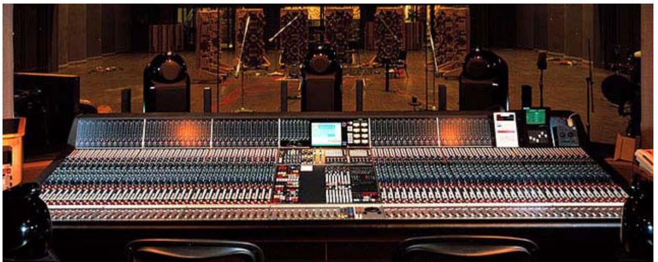
The 88RS at Skywalker Sound in California
