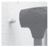
Once the holes have been drilled, place the wedge anchor into the hole. Using a hammer, gently tap into place.
