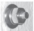
Correctly seated wedge anchor bolt.
