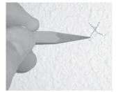
Once the stud has been located, use a pencil to mark the center of the stud.
