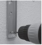
Use a drill and a 1/8" drill bit to pre-drill the mounting holes.
