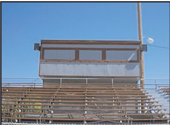
Loudspeakers Installed on Press Box
