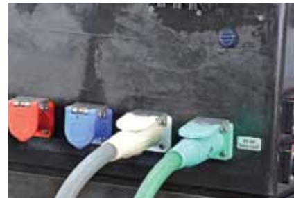
2. Insert the Cam connector into the receptacle and rotate Cam connector at least 90 clockwise degrees to lock
