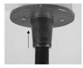
Slide plastic cap up to cover the bolt.
